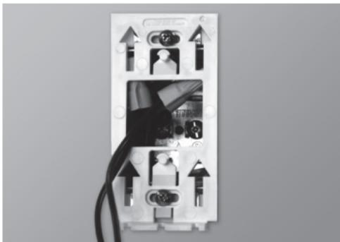
8. Align the little slots located on the top of the thermostat with those on the the mounting base and secure the thermostat to the mounting base. Note that you can also position the thermostat on the left or the right side of the junction box (see the illustrations below). Then, tighten the screw at the bottom of the unit.
